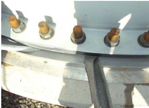
PU-foam used as temporary form
