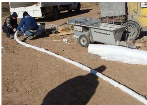
Reflective installation being applied to the hoses
