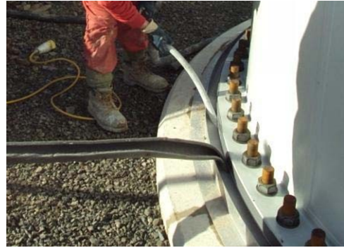
PU-foam used as temporary form
