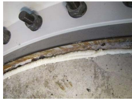
Pumping Masterflow 9300 underneath the flange of the tower
