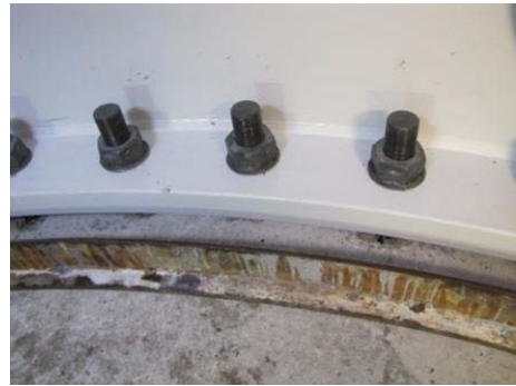
Steel formwork installed on the inside
