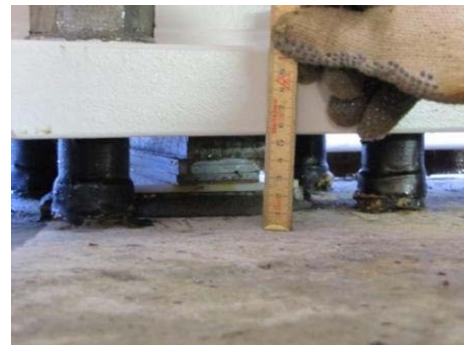
Situation after installation of tower base.
